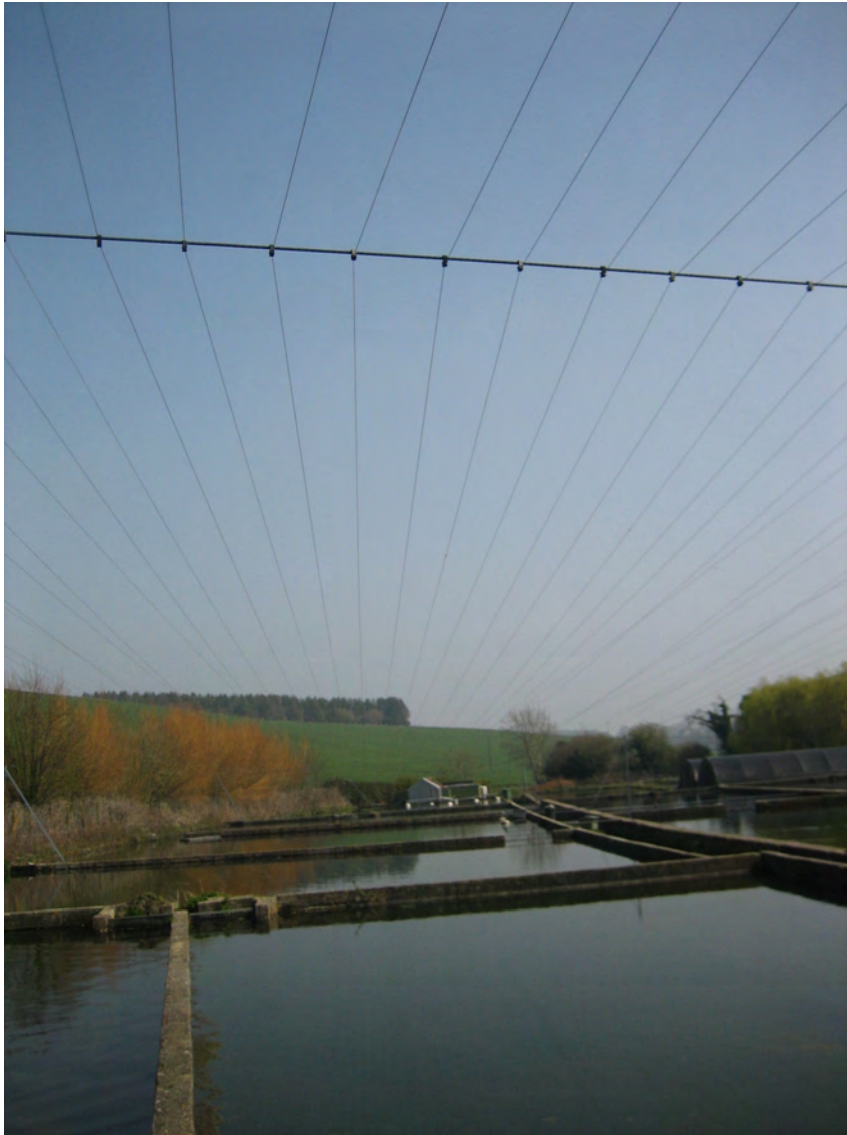
Figure 11 – Heron wire at Houghton Springs Fish Farm.
